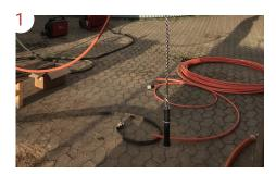
A cable mole with cable sock is mounted at the end of the cable. Two sponges (with lubrication in the middle) are the first thing to insert in the 40 mm duct, which is connected to the Y-block. After lubrication, the cable mole is inserted in the duct.
