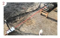
The sponges are the first thing to blow through the duct. This cleans the installed duct and controls that the sponges arrive at the opposite end of the duct. After the sponges arrive, the fiber blowing can commence. Start applying 1-2 bar pressure to straighten out cable mole and cable sock.
