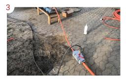
Approximately 50 m into the fiber blowing process, the micro cable meets a bit of resistance making the cable wobble. To avoid this, the air supply to the Y-block was increased. This destresses the cable, which stops wobbling.
